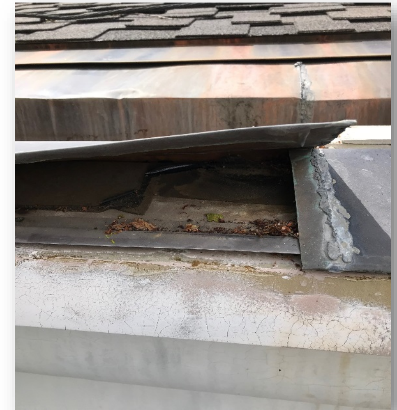
Copper gutter coming apart at the seam, allowing water to penetrate the roof eave.
