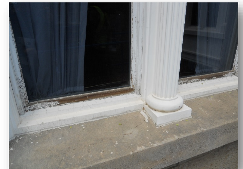
Typical condition at wood and fiberglass windows. Paint has worn away at wood window sills, note the fiberglass is in good condition with only cracking and peeling of paint.
