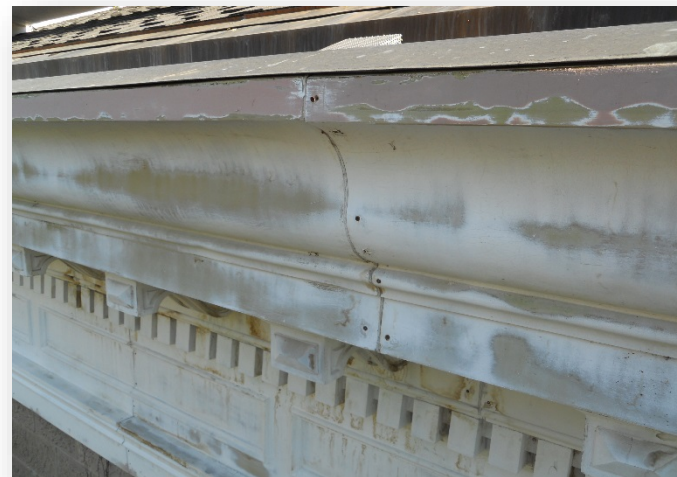
Worn away paint on the fiberglass panels.
