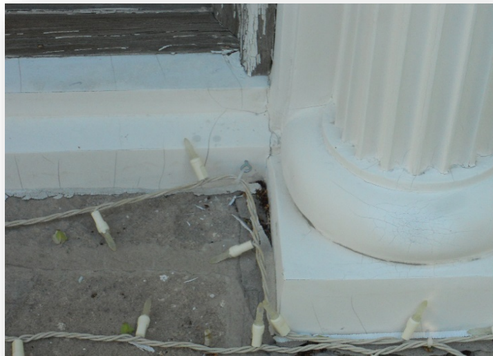
Eye hook inserted into fiberglass frame for hanging of Christmas lights. Also notice the deteriorated wood frame of the window versus the fiberglass frame of the window.
