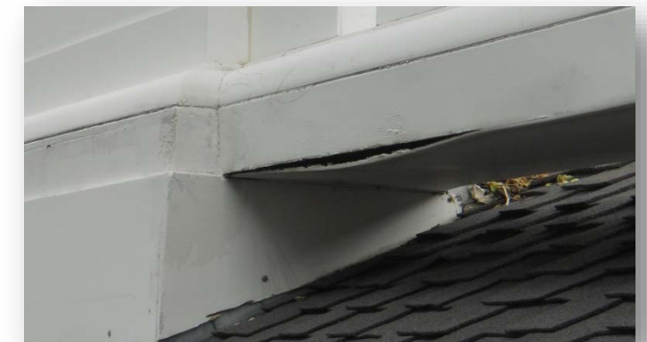
Large tear in fiberglass balustrade at horizontal and vertical edge.
