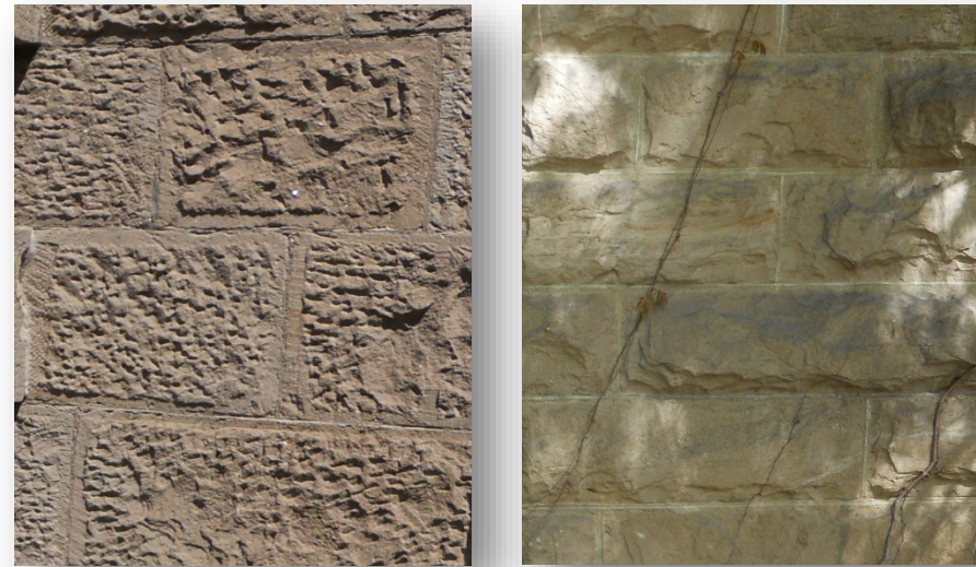
Capitol Building masonry versus Annex Building masonry
