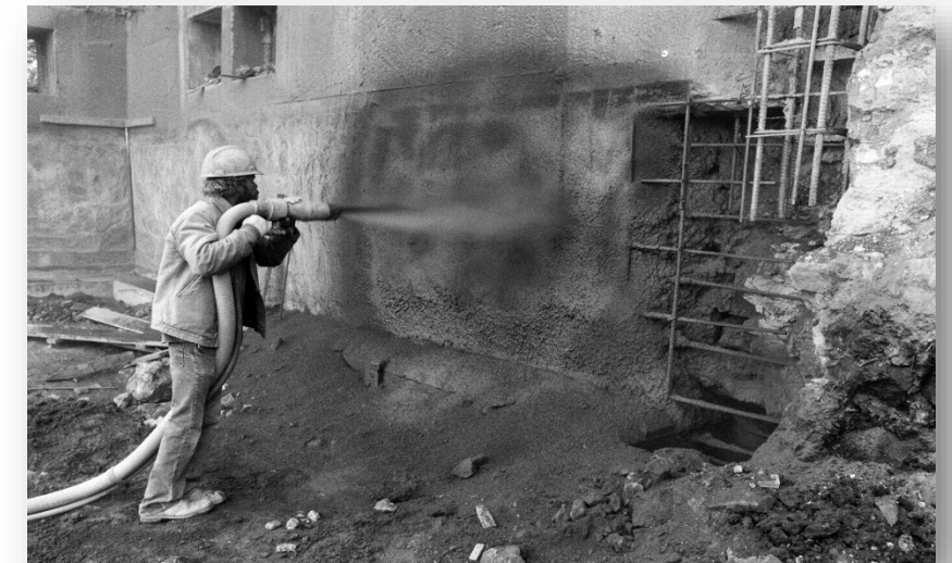
Shotcrete and rebar applied to the backside of the sandstone masonry veneer, 1978-1979 rehabilitation project.
