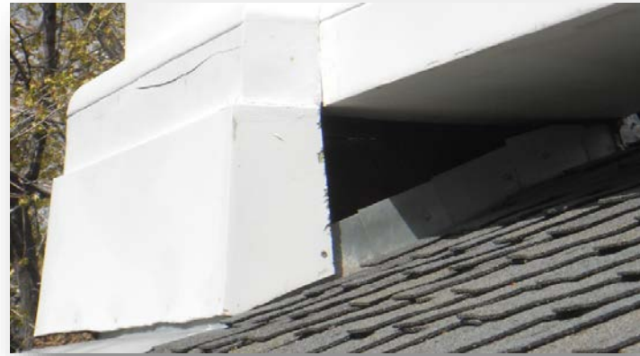
Missing base piece of balustrade. Potential nesting place for birds and vermin.
