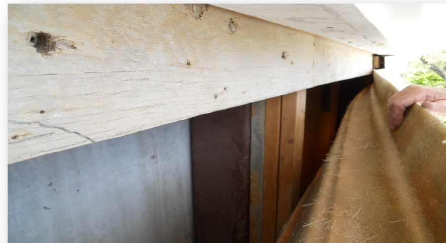
Fiberglass sub-structure at entablature: plywood attached to built-up 2x4s attached to a metal structure. Notice the concrete staining on the 2x4 and the plywood is also concrete stained as if it were a form board.
