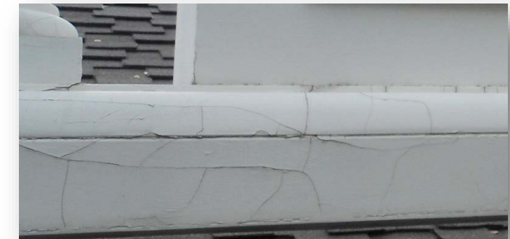
Cracking paint on the fiberglass substrate.
