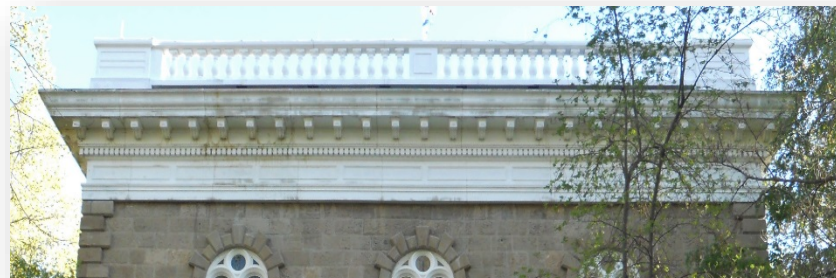
The use of fiberglass from the entablature to the roof balustrades.
