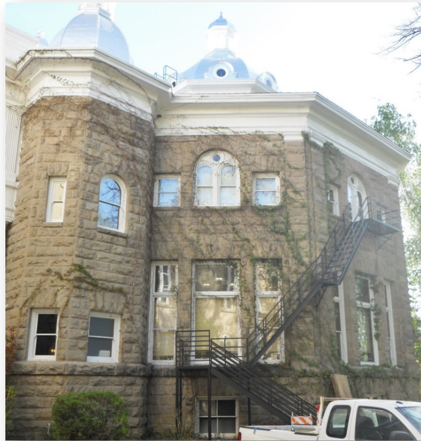
Vine growth on the Capitol Annex.
