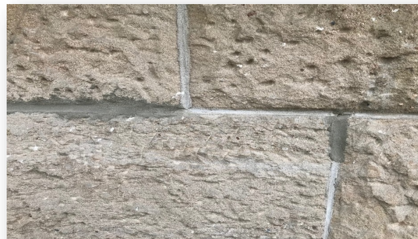
The dark gray mortar (vertical joint) is a repair while the light, thin line of mortar is the oxidation from the original white lead tuck-pointing. This particular grout joint on the Capitol Building tested positive for lead, thus confirming the use of white lead oxide.
