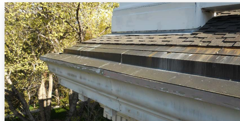
Typical copper gutter at the roof eave of the Capitol Building with brown patina which is most common in a dry desert environment.
