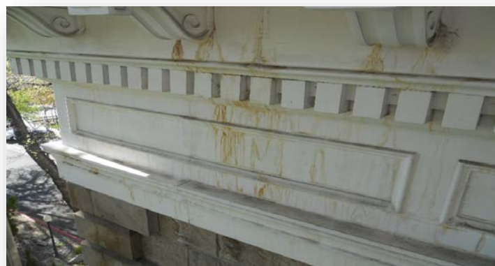
Staining on the fiberglass entablature, a sign of water intrusion from above.
