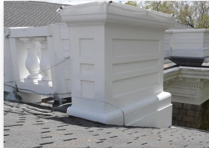
Rope lighting fastened to the top of the balustrade.
