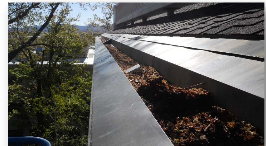
Copper gutter filled with dirt and debris.
